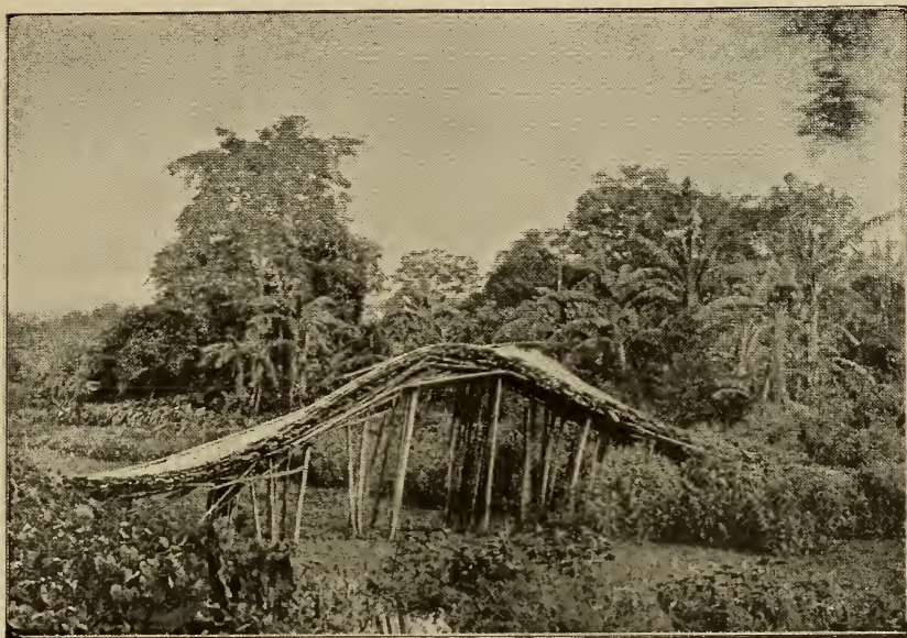
FIG. 1. BRIDGE OVER STREAM AT RANGPUR.
