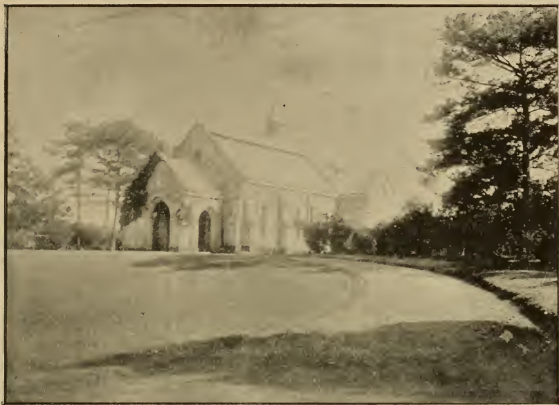
FIG. 1. ALL SAINTS CHURCH, SHILLONG. Before the earthquake (Cf. Pl. I.)
