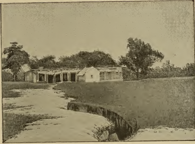
FIG. 1. FISSURE IN COMPOUND OF JUDGE'S HOUSE, RANGPUR.
