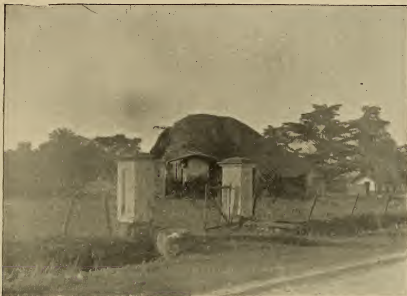
FIG. 1. GATE PILLARS OF TELEGRAPH SIGNALLERS' QUARTERS, GAUHATI.
